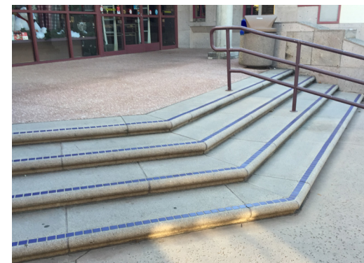
concrete stairs with tile accents on treads
