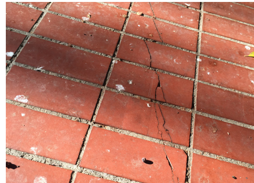
mortar set brick on concrete slab
