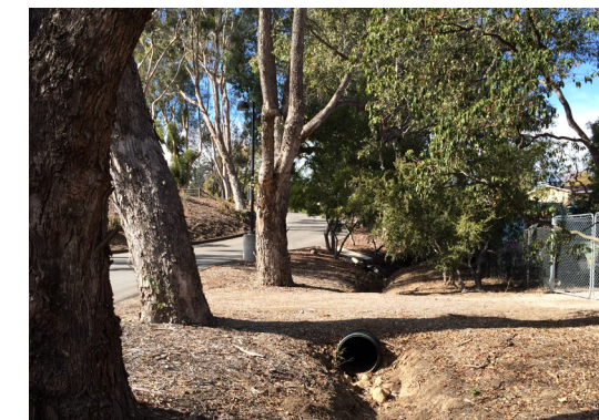
drainage ditch along northern edge of campus
