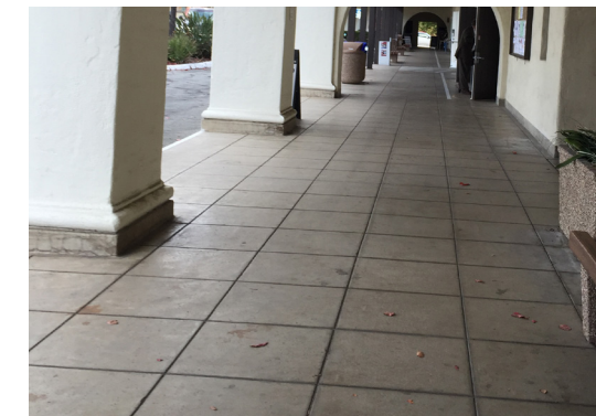
concrete arcade walk
