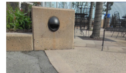
Pathway material transition; abrupt change in level and hazardous surface features
