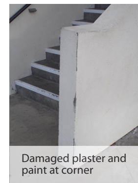
Exterior walls, peeling plaster paint
