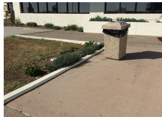
construction joint with sealant between concrete with exposed aggregate and concrete with integral color
